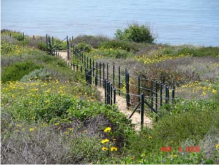
Current condition of trail and trail fencing.
